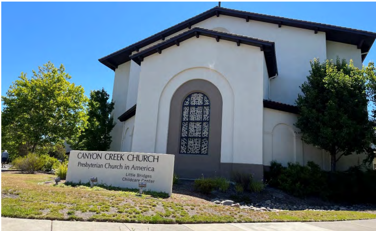
Figure 3.1-8 View 6: Looking southeast toward Canyon Creek Presbyterian Church from intersection of Gale Ridge Road and Bollinger Canyon Road
